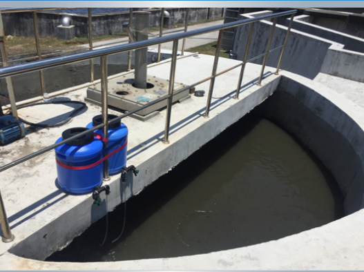
➔ Simple drip feed application Dose: 40 Litres per day
