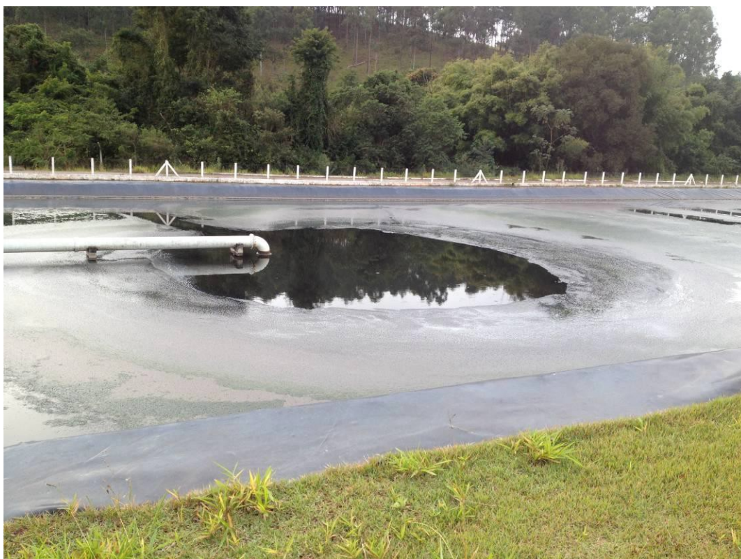
Figure 1: View of maturation lagoon No. 2, depicting the degree of aggradation prior to the application of Biocelerator
